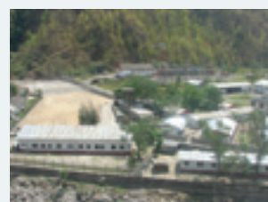
Khimti 1 power house and complex
