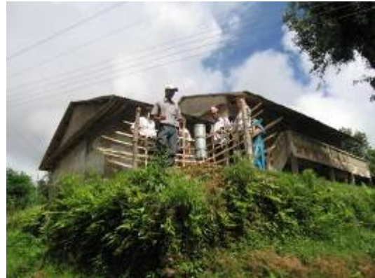
Figure 2.13: Installation of raingauge at Kauli
