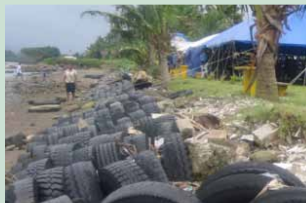
Coastal protection structures in Lami, Fiji © UN-Habitat
