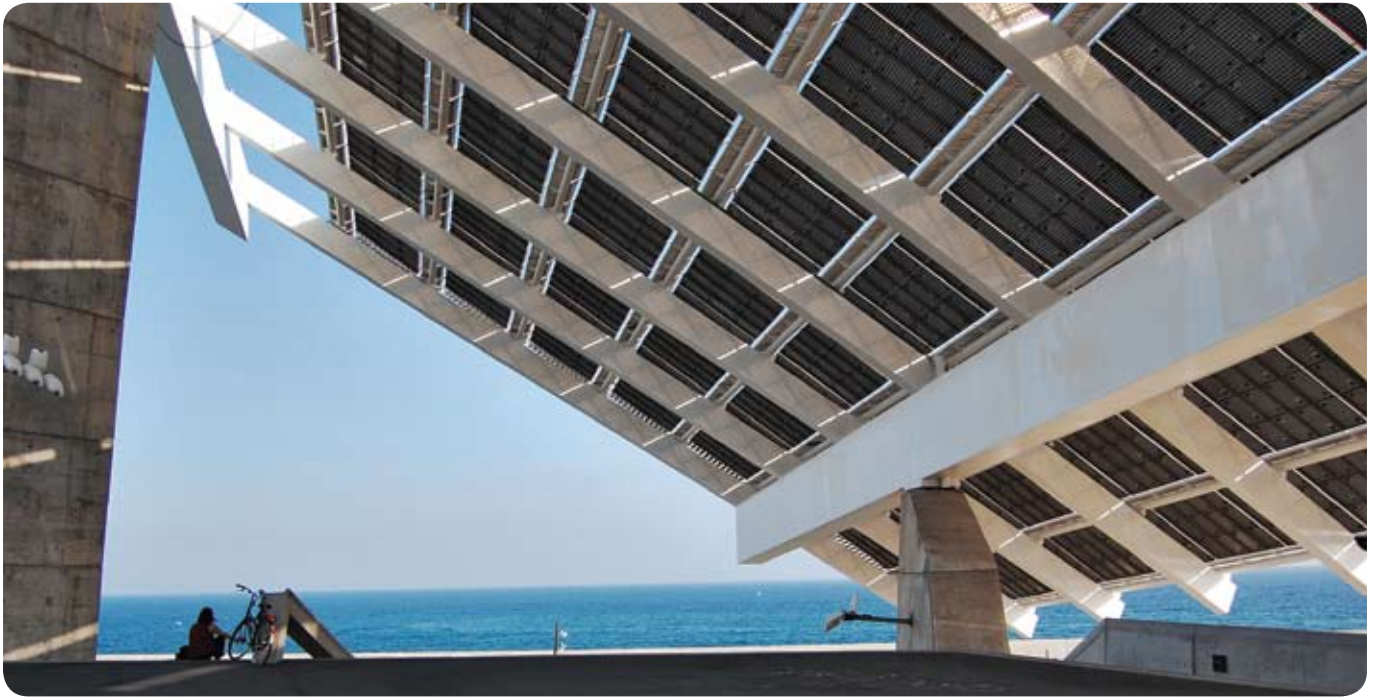
Esplanade and Photovoltaic Power Plant by racEcar_yayas/flickr.com
