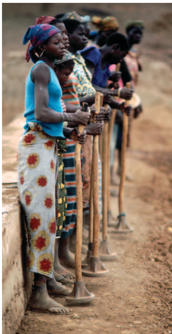
Women work to pound and terrace the soil in drought-stricken Burkina Faso to control erosion and manage water in the rainy season
