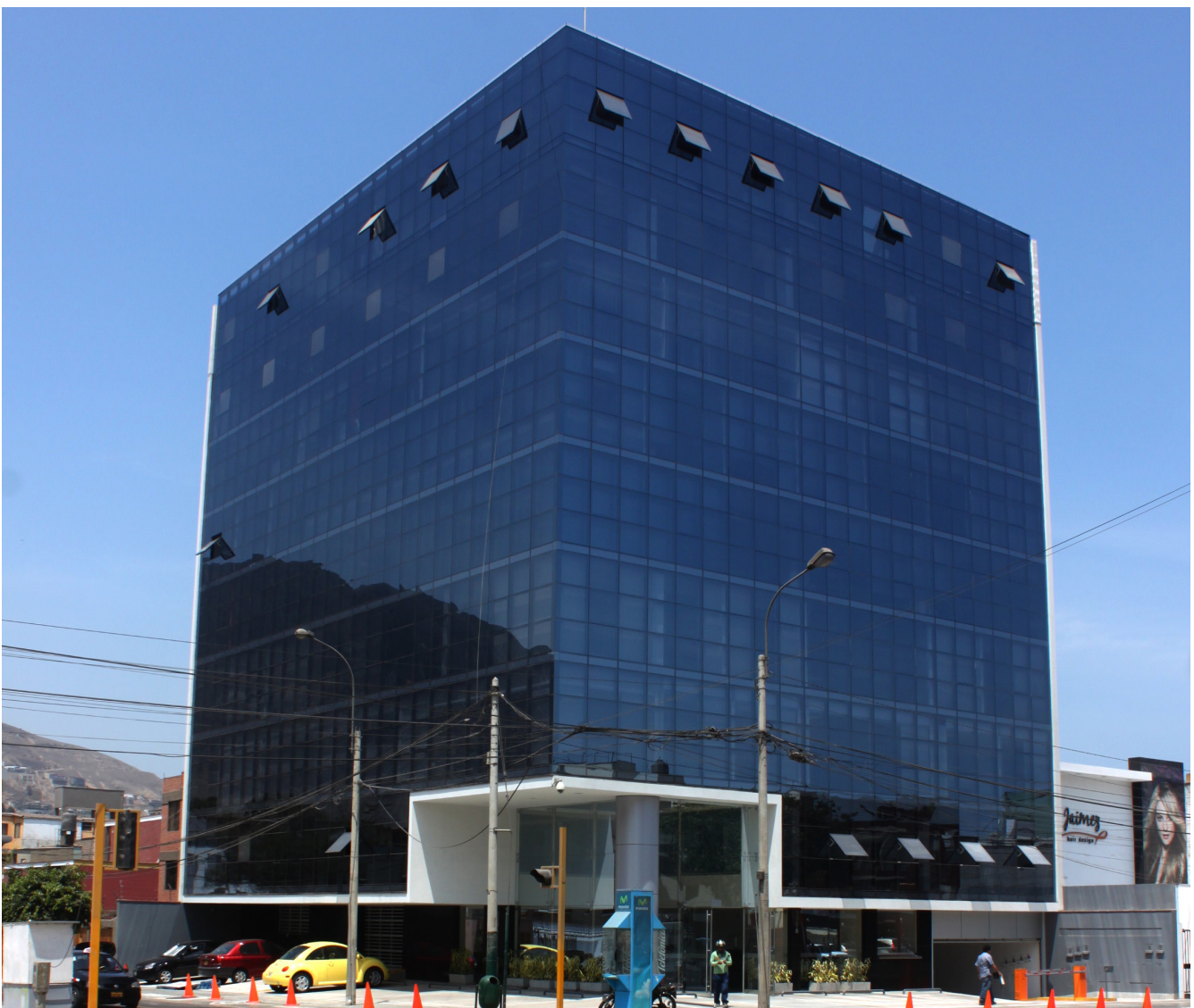
Johnson Controls Offices - LEED Certified (Source: Peru GBC)
