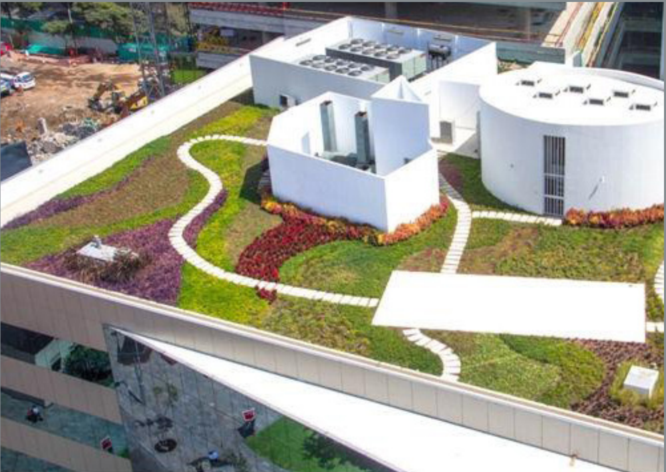
Figure 6.2 Green Roof of the Real Seis Building of the Entrepreneurial Center of Real de San Isidro (Terra, 2013).
