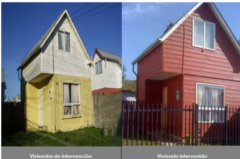
Housing before and after thermal conditioning. one of the Program grants Homestead Protection (Source: serviumagallanes.cl)
