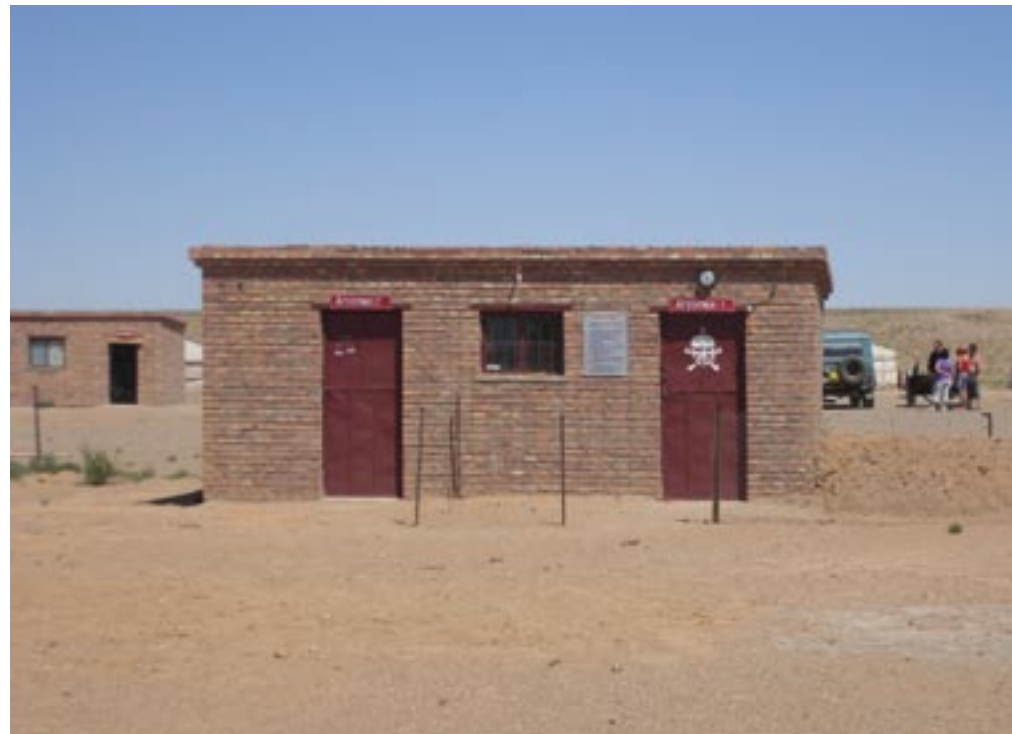
Informal gold ore processing plant, Khongor Soum, Mongolia
