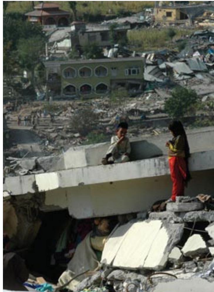
Children sit amidst the rubble of their home in Balakot, Pakistan in 2005. Hazard contingency plans are part of the re-building exercise
