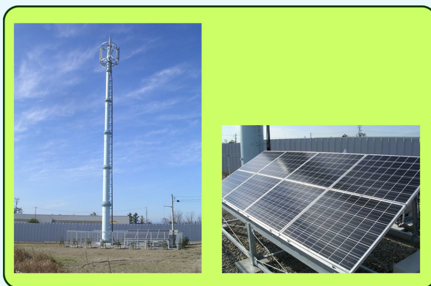
Figure 6.4 – Equipment installed for tribrid technology field trials
