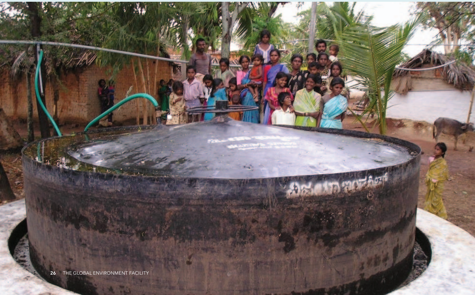
Group biogas plant to provide clean cooking gas, Biomass Energy for Rural India Project
