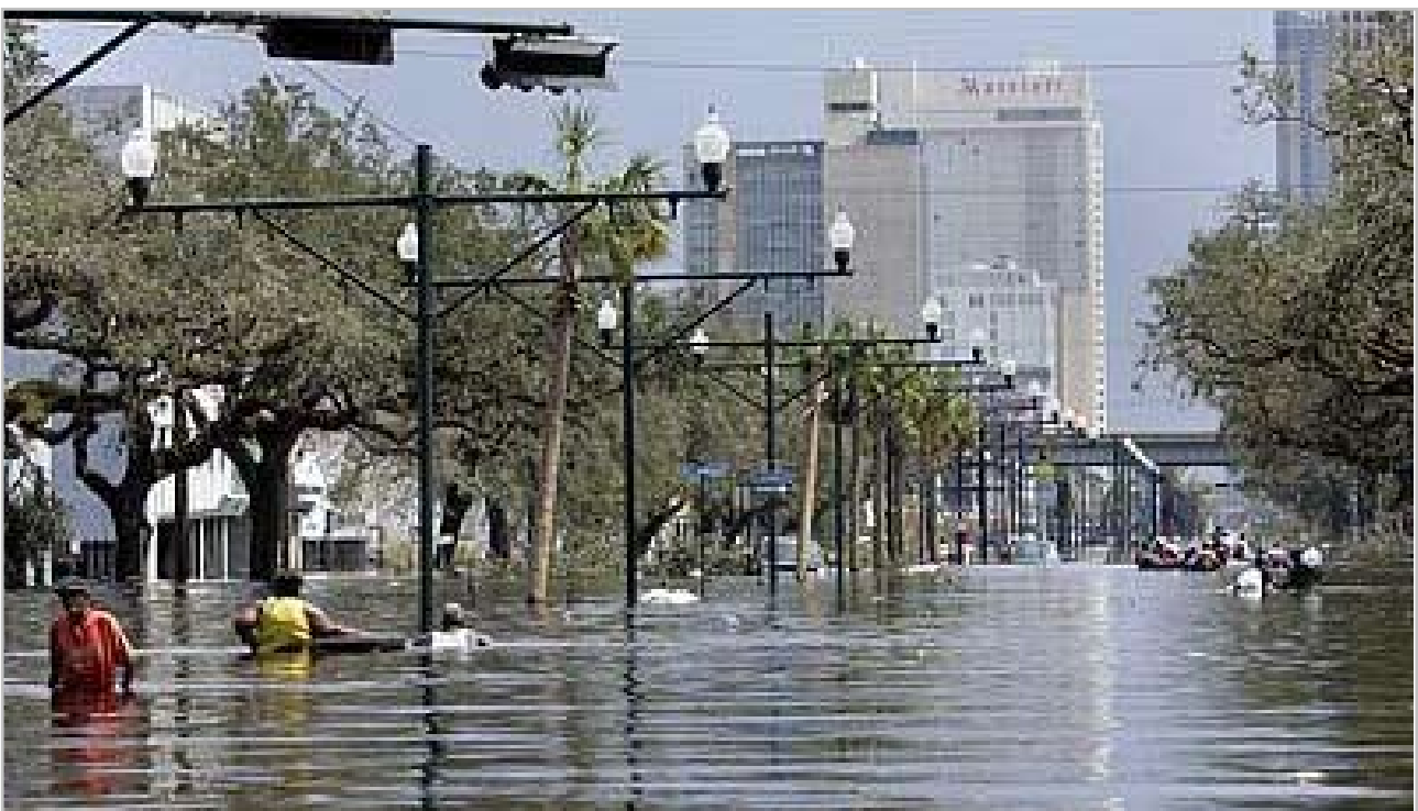
Canal Street, New Orleans, after hurricane Katrina, 2005
