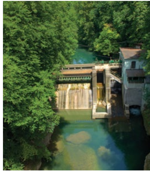
Fig. 3.1.9. Small hydropower plant on the Kokra river (Slovenia).
