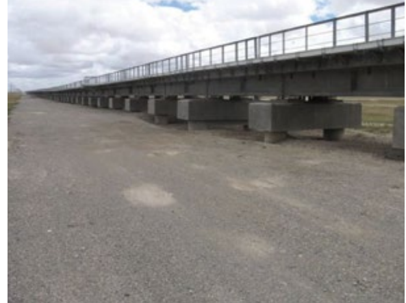
Fig. 2.8.14. Road standing on supports sunk deep into the ground.
