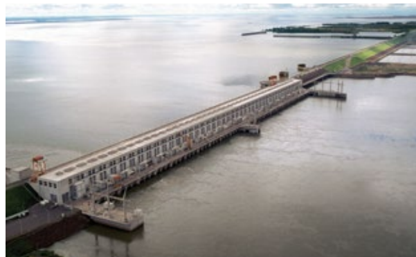
Fig. 3.1.11. Yacyreta Dam on the Parana river (Paraguay, Argentina)
