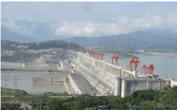
Fig. 3.1.10. Three Gorges hydropower plant (China).
