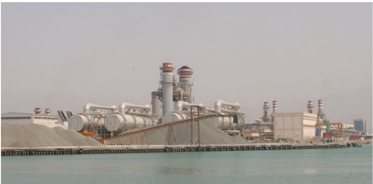
Fig. 2.4.9. A seawater desalination plant in the United Arab Emirates.
