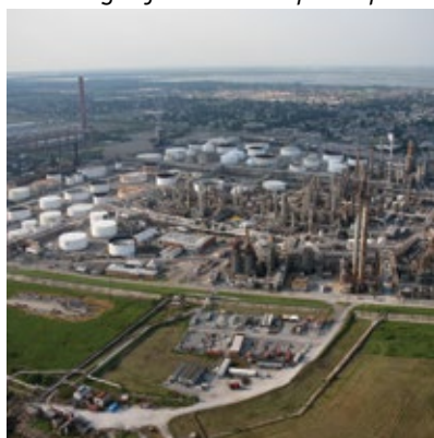
Natural gas-fired thermal power plant.
