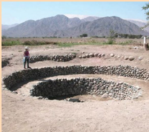
Fig. 2.4.10. Water collection system in Nazca regions (southern coast of Peru) for underground aqueducts and distribution of groundwater.
