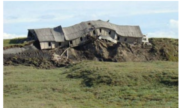
Fig. 2.8.9. A building destroyed by uneven bulging and subsidence above permafrost.
