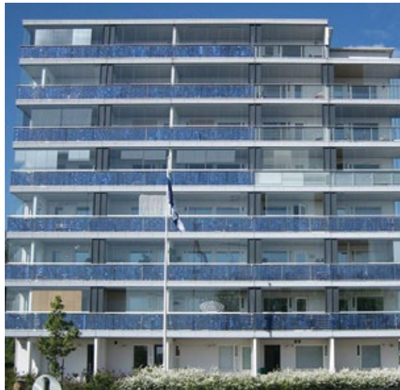
Fig.3.2.12. A number of low-energy buildings have been constructed in the Viikki district of Helsinki (Finland). Panels that store energy from the sun have been built into the facades.
