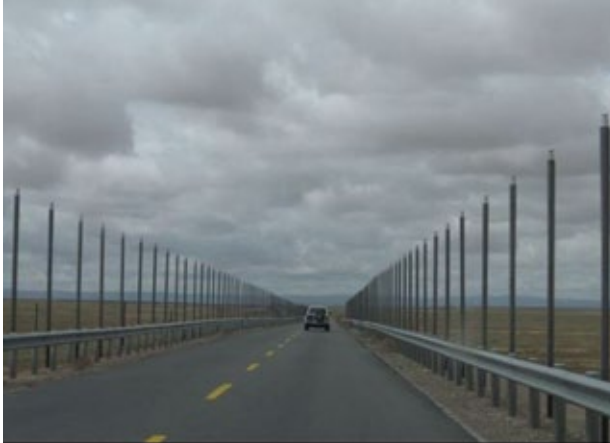
Fig. 2.8.13. Road with soil-freezing thermosiphons.
